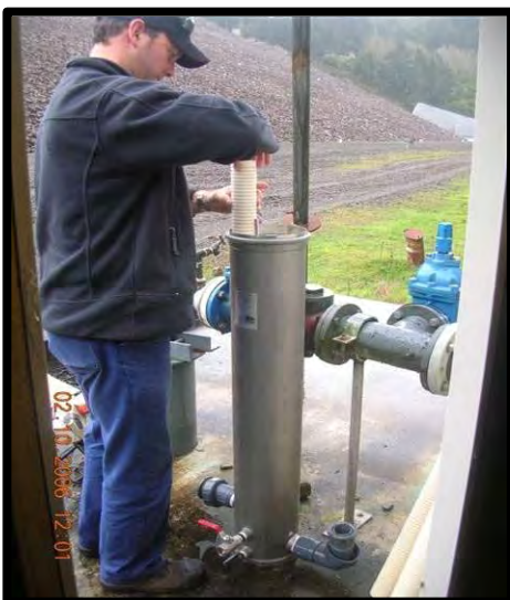
Figure 6: Changing a cartridge filter
