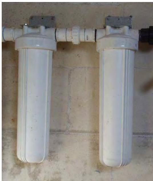
Figure 1: Coarse pre-treatment cartridge filter mounted before a fine cartridge filter
